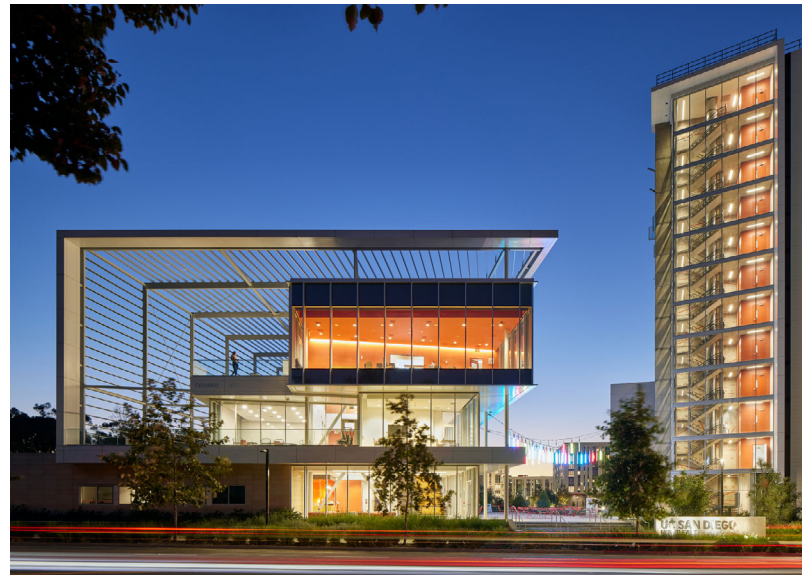
UC San Diego Nuevo East Graduate Student Housing, Design-Build by Hensel Phelps | Mithun, Photo by Bruce Damonte
