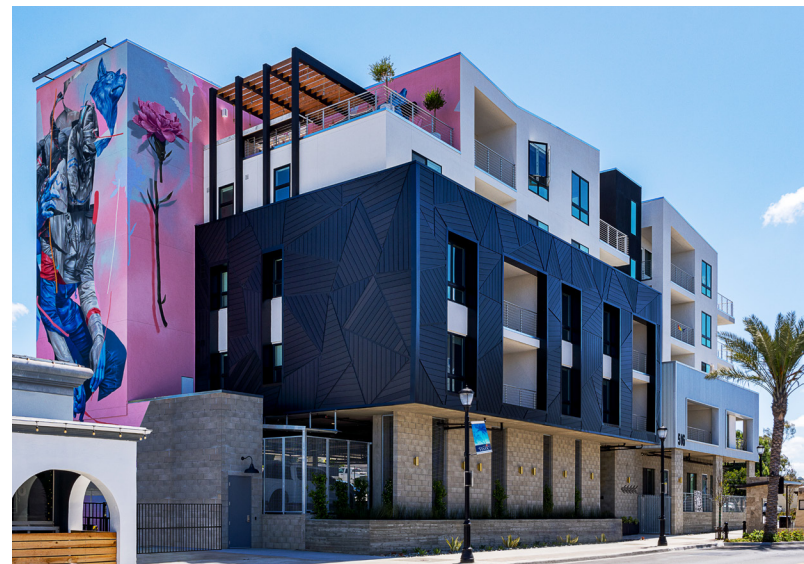
Found Lofts, Developer: Tideline Partners, Stephen Dalton Architects, Photography: Fernando Phillipi Orchid Award-winner/SD Architectural Foundation
