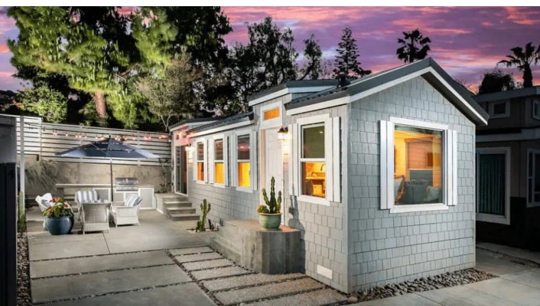
Accessory Dwelling Unit (ADU) by Backyard Homes as seen in Coast News April 5, 2021
